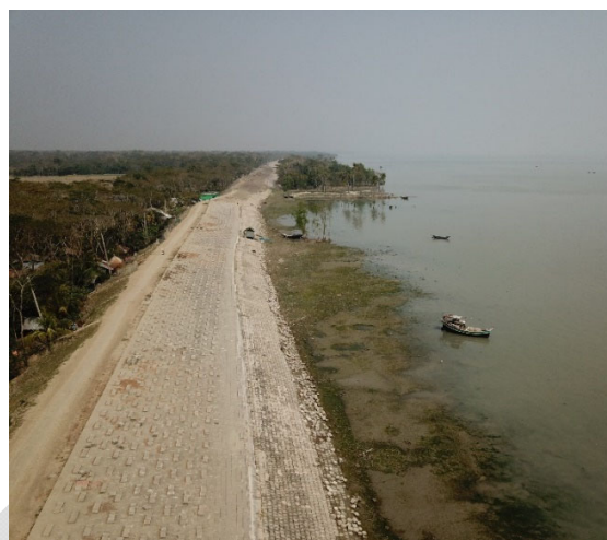
Figure 2.5: Embankment slope protection works in polder 35/1
