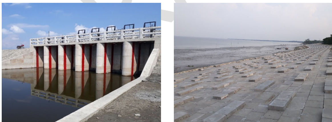
Figure 1.3: Sluices and slope protection works under CEIP-1
