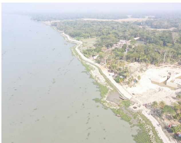
Figure 2.4: Erosive banks of polder 39/2C and bank protection works by CEIP-1
