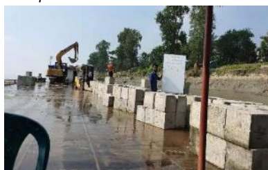
Dumping of CC blocks for bank protection works under CEIP-1
